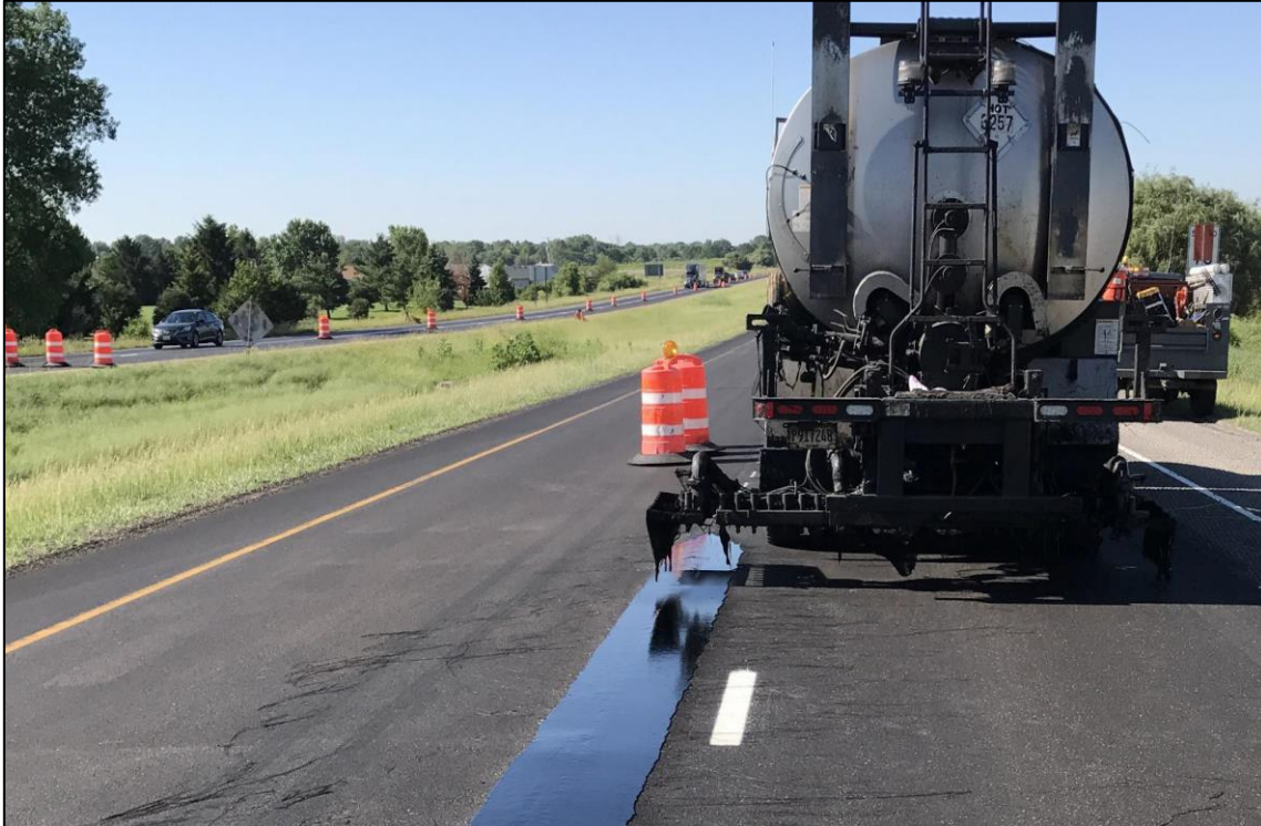
Void Reducing Asphalt Membrane (VRAM)
