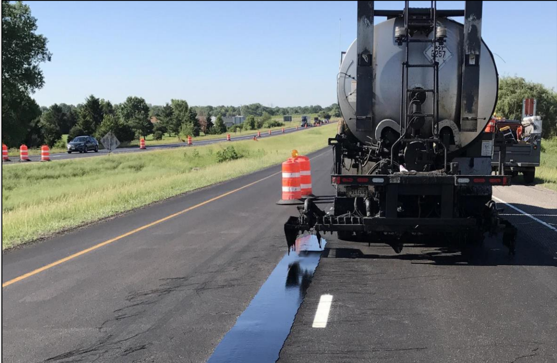
Void Reducing Asphalt Membrane (VRAM)
