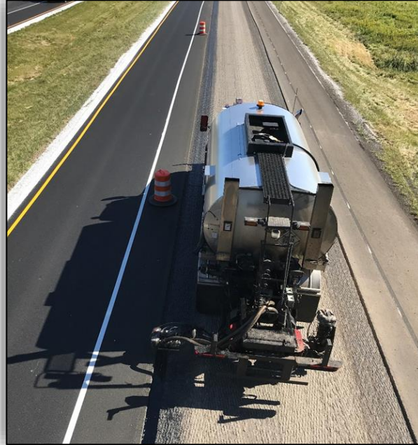
18" wide VRAM application or 9" wide mill and fill
