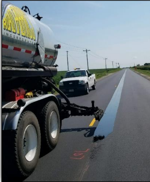
18" wide VRAM application or 9" wide mill and fill
