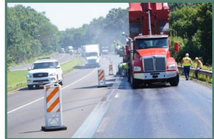
PennDOT District 1, I-80
