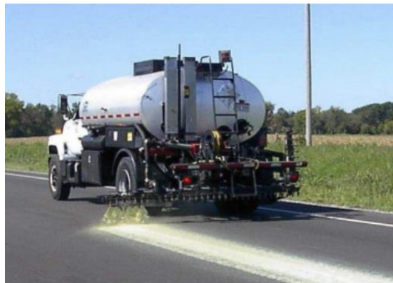
Calvert. Fog Seal Application of Rejuvenators and Seal Coats.
