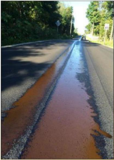
RPE used as a longitudinal joint preventative treatment immediately following application (left), after penetrating joint (center), and after cure (right).
