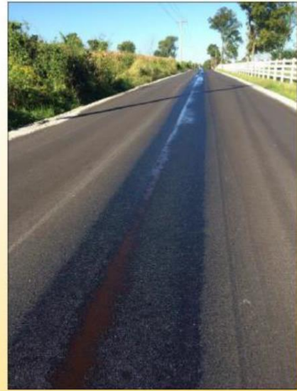
RPE used as a longitudinal joint preventative treatment immediately following application (left), after penetrating joint (center), and after cure (right).
