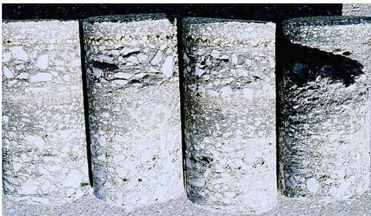
Figure 7. Cores from an Asphalt Pavement Showing Moisture Damage in a Near-Surface Layer.
